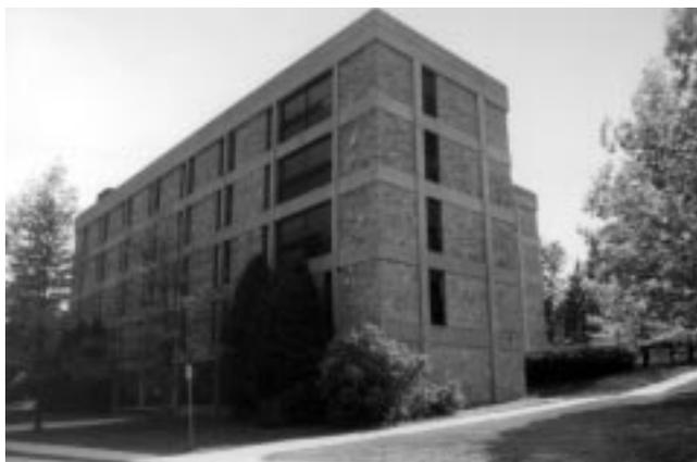
An onsite “crusher” is grinding the 35-year-old science center’s 600 tons of concrete into project fill to be used for the new library construction and on roads. Limestone exterior walls will be salvaged for reuse, and copper, steel, aluminum, glass and wood will be recycled. Much of the center’s old science equipment has already been donated to schools in Vermont and New Hampshire.
