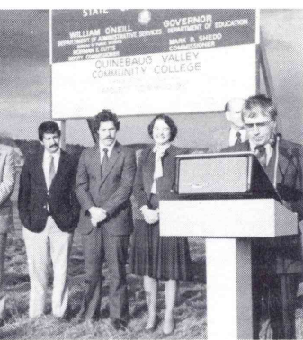
Miller speaks at groundbreaking,
