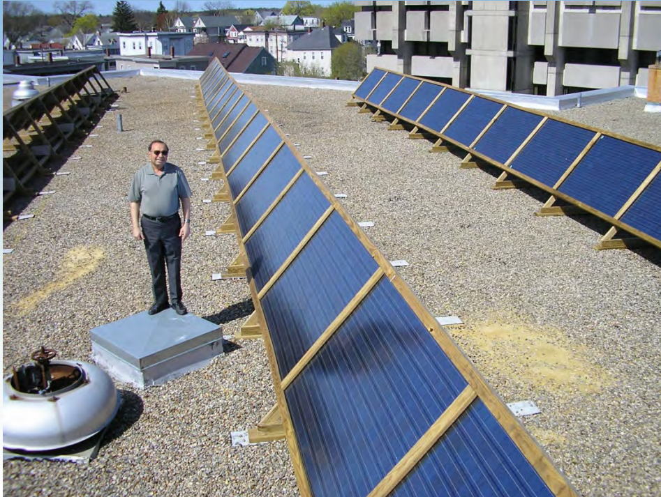
Umass Lowell 10.56 kw, installed with students
